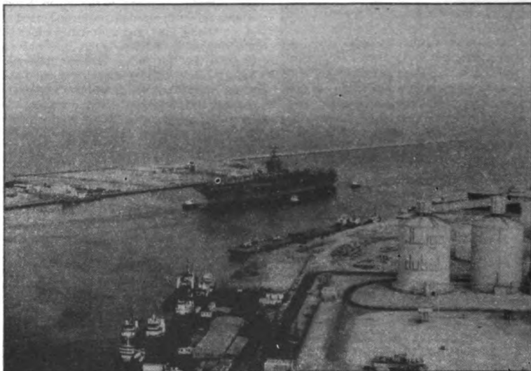
EXCELLENT PORT FACILITIES AT JEBEL ALI
